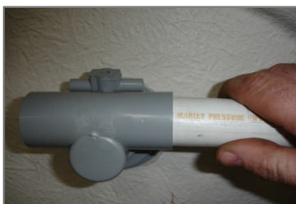
Glue 25 pressure pipe into sockets
