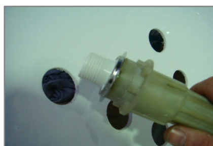
Locate retainer and mounting flange into hole in bath
