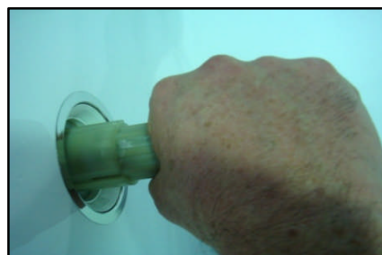
Using Installation tool screw retainer into jet body. Hand tighten only DO NOT OVERTIGHTEN
