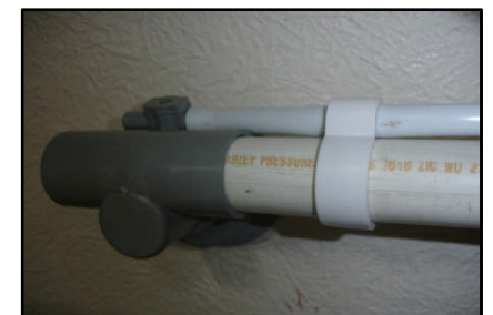
Fit clamping clip to retain pipe
