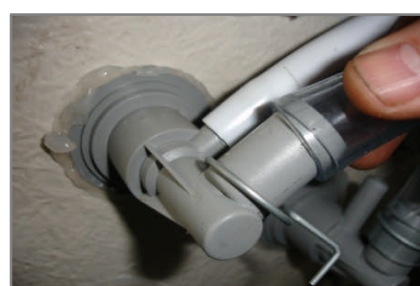
Push 19mm flex pipe on barb spigot.
