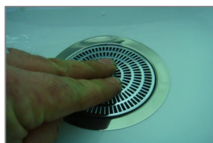
CHECK THAT THE EDGE OF THE MOUNTING FLANGE IS PULLED DOWN AND THERE IS NO SHARP EDGE
