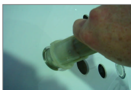
Using Installation tool screw retainer into jet body. Hand tighten only DO NOT OVERTIGHTEN
