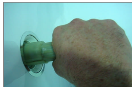
Using Tool MT0168 tighten retainer into elbow. Max torque 14nm
