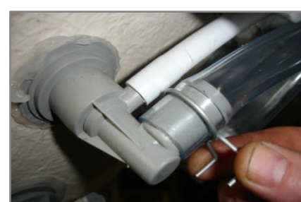
Fit clamping clip to retain pipe
