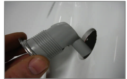
Remove nut from body and pass body through hole in bath.
