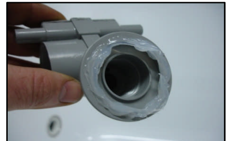
Apply an adequate amount of silicone to front flange of body
