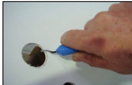
THERE MUST BE NO BURR ON EDGE OF HOLE, a burr could stop the mounting flange sitting down flush
