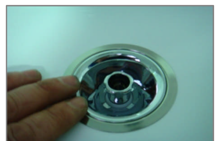
Check jet is sitting flush with mounting flange.
